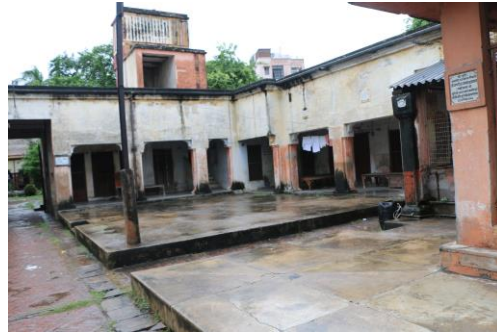
Mumukshu Bhawan At Asi
