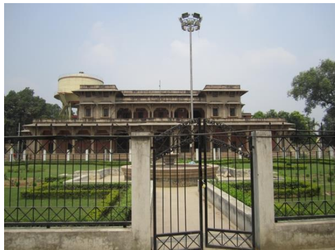
The Saraswati Bhawan Library building, SSU (Photo source: official website of SSU)
